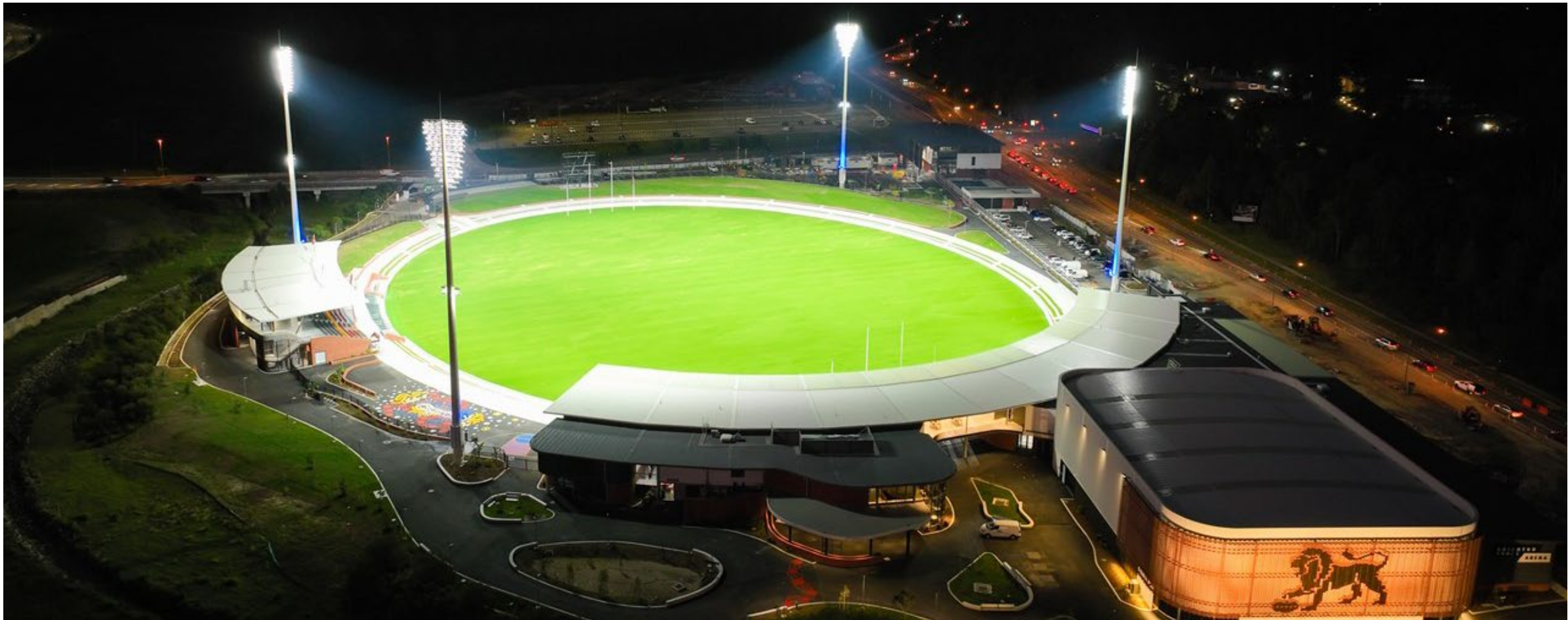
Brisbane Lions Training and Administration Facility Springfield Central QLD, Australia
