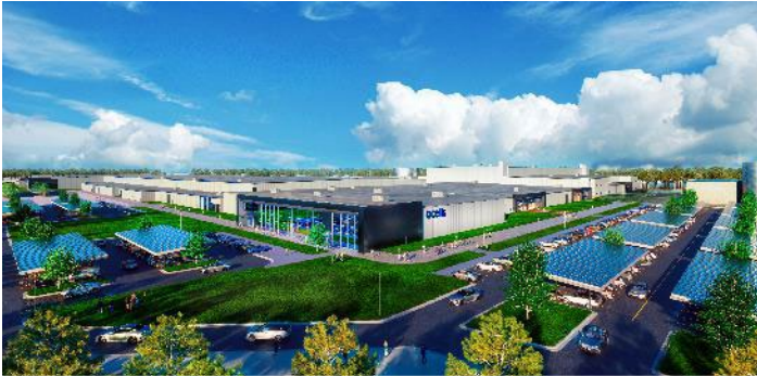
Q-Cells Solar Power Manufacturing Facility
